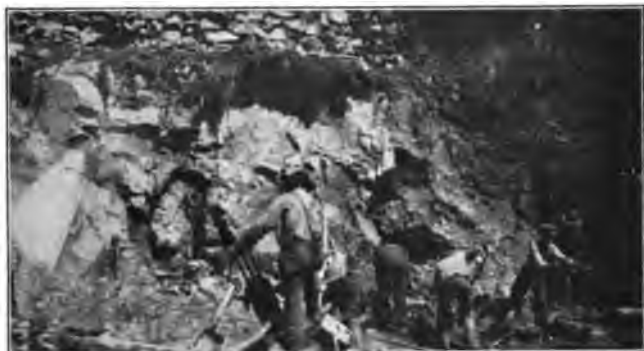
B. STARTING EXCAVATION AT SOUTH LAKE MINE.
